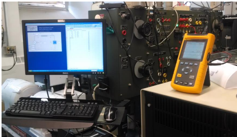
Figure 49. Utility feed measurements
