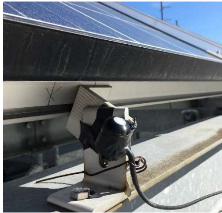
Fig. 9. Irradiance sensor mounted.
