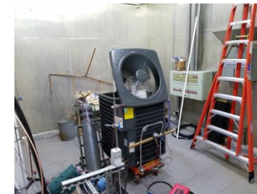
Air-source heat pump outdoor unit being installed
