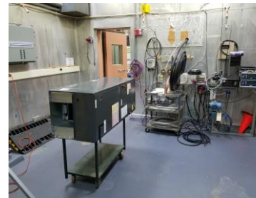
Air-source heat pump indoor unit being installed
